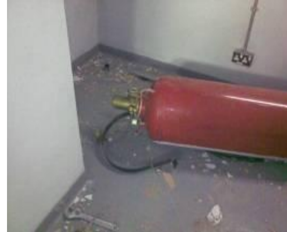
Damaged FM200 Cylinder
